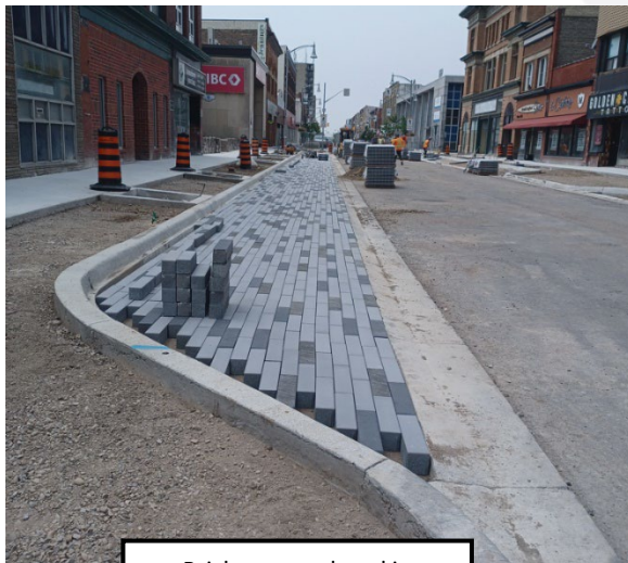
Brick pavers placed in parking lay-by
